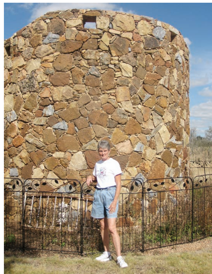
Karen Wilkens is pictured in front of the 10,000 gallon cistern she and her husband Joe first envisioned after seeing a similar one on a trip to Italy and Greece. Inside the rock façade is a fiberglass tank surrounded by cinder blocks, mortar and rebar.
